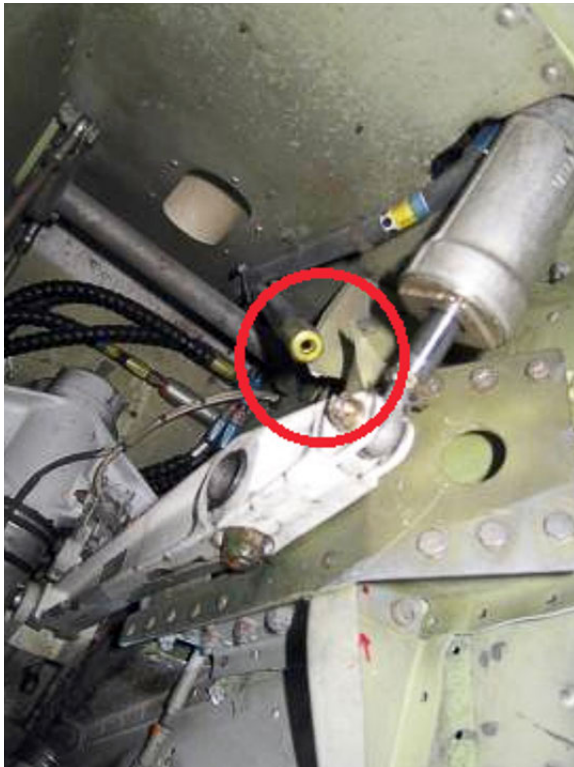
Figure 6. Return of the hydraulic line that supplies the actuator
